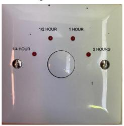
turns the system on and subsequent pushes advance the time as shown, a fifth push switches the system off – there will be a short delay before it can be turned on again as the system resets itself. The system will shut off automatically after the set time unless you reset it. The heating is usually on from 1 October until 30 April.
